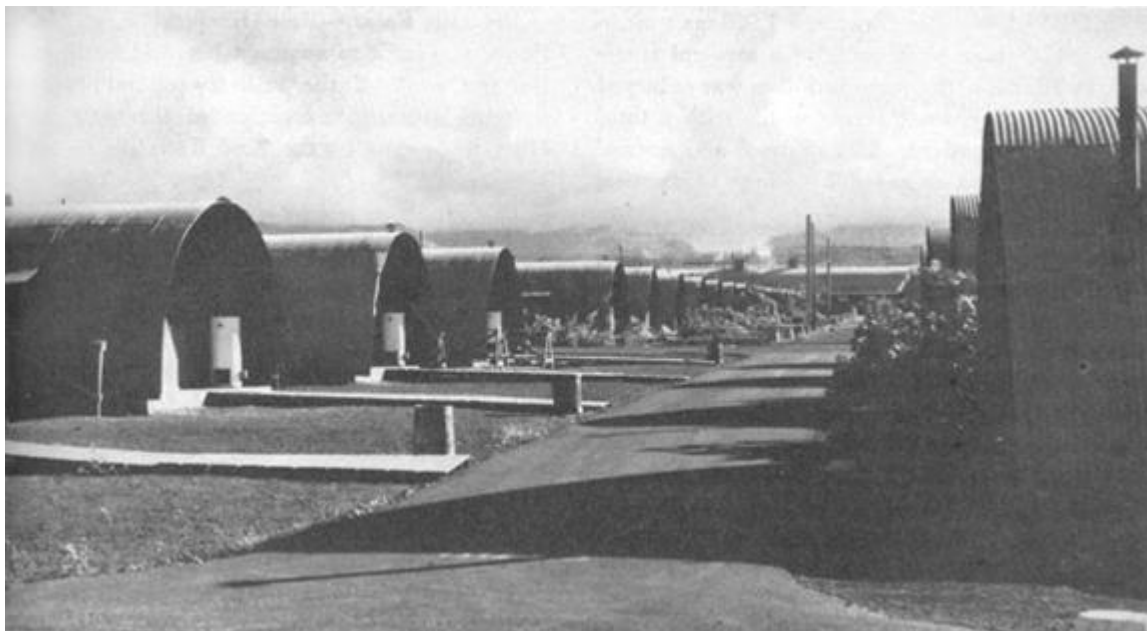
Wards at the Naval Hospital on Moanalua Ridge
