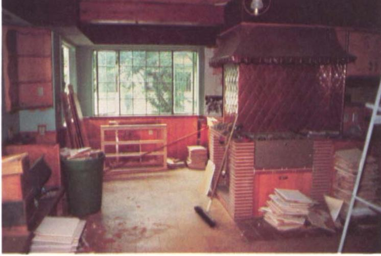
The kitchen (above), which had been Early-Americanized in the 1950s—knotty-pine cabinets and trim, scalloped copper work and an island range—had to be completely gutted. The window area where the sink stood was removed and the wall there filled in (right), and treated between the tops of the cabinets and the header strip with subway tiles.
