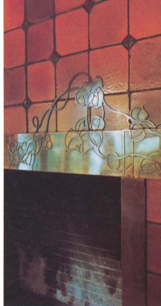
**A copper header with trailing-vine overlay conceals rebar holes above the fireplace lintel.**
