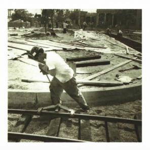
Left: Construction of trackage for the Main Street Horse-Drawn Streetcars is under way in spring 1955 at Disneyland; here, the teardrop loop at Main Street Station is being assembled. In the foreground, a worker applies muscle power to a rail-bending device, straightening out a kink in the curve prior to spiking the rails in place on the wood crossties. Roger Broggie photo, © Disney Enterprises, Inc.
