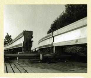
This moveable section of beamway, behind Tomorrowland, allows Monorail trains to be switched from the main line (left) to the "Roundhouse spur." Both, © Disney Enterprises, Inc.
