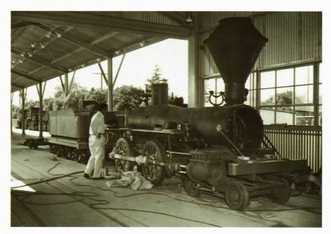
Top: Inside the Disneyland "Roundhouse" facility (actually a rectangular building), assembly of locomotives Nos. 1 and 2 is well along in early 1955. The Dixon-built boilers are going into place atop the Wilmington Iron frames; note the heavy duty machine tools at right, along the wall. CPHS collection, © Disney Enterprises, Inc.
