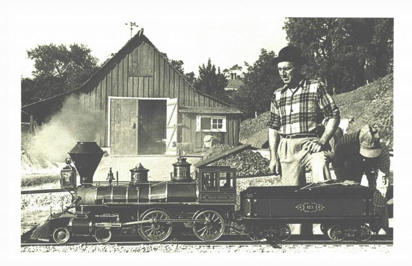
equipped with four spoked wheels—had been meticulously fashioned from hand-drilled brass and then riveted together. The tender held three-and-one-half gallons of water, and was equipped with a pump to supply water to the locomotive's boiler through a connecting line.
