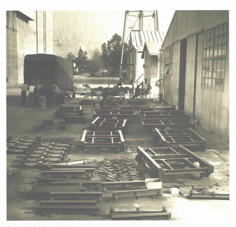
Frames, springs, brake shoes and rigging components, and wheelsets are being assembled into trucks at the Disney studios, circa early 1955. Soon, they will be completed and installed under the passenger coaches, themselves under construction in a nearby sound stage. Roger Broggie photo, Ward Kimball collection, © Disney Enterprises, Inc.
