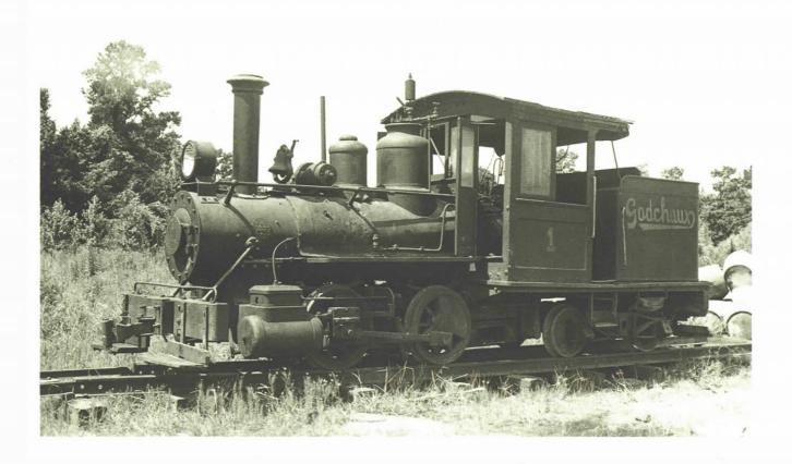
cylinders, and domes appeared sound, along with the valves and levers on the boiler's backhead (inside the cab). Jerry tried the industrial engine's bell, and it rang true even though it was caked with road grime and coal soot. He then wiped away the dirt covering the solid brass builder's plate, which read: Baldwin Locomotive Works-Philadelphia-1894-No. 14065.
