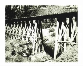
Above: Unanticipated delays and expenses were incurred by Walt during planning and erection of this impressive wooden trestle. Its height—crossing nine feet above a lower level of track—subjected the 46-foot-long scale-model structure to costly public construction standards. Steve Booth photo.
