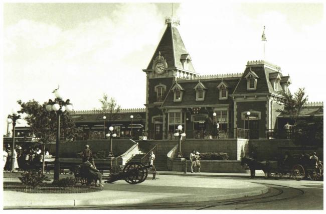
third-floor dormers—to create an illusion of height. The facia features brick and cut stone, with wooden framing around the doors and windows. Wrought-iron filigree accents the main building's roof line, and that of the platform wings; roofing shingles depict three different designs. Two huge clocks show their faces, one toward the tracks and the other toward Main Street.
