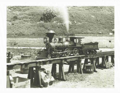
Ready for a run, the Lilly Belle is "popping off" as the boiler's safety valve releases excess pressure. The little trestle in the view is the "ready track," located in the Yensid Valley's rail yard. Here, the locomotive and rolling stock were easily worked on; the elevated track allowed unrestricted access.
