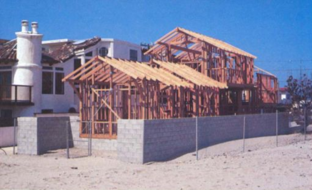
Framing, plain and fancy. The floors and walls for this California beach house are conventional 2x framing (above), except for purlins that extend the top plates of the long exterior walls. These 6x6s are supported with Craftsman-style knee braces. The concrete-block foundation walls were laid up flush with the wood framing and later plastered as a continuous surface. The king-post truss that separates the family room from the living room (below), combines wood joinery and metal fasteners in a design that's both handcrafted and practical. The tops of the two posts are tenoned to form seats for the bottom chords, and the king post and web members are also tenoned on both ends where they are sandwiched between the double chords.
