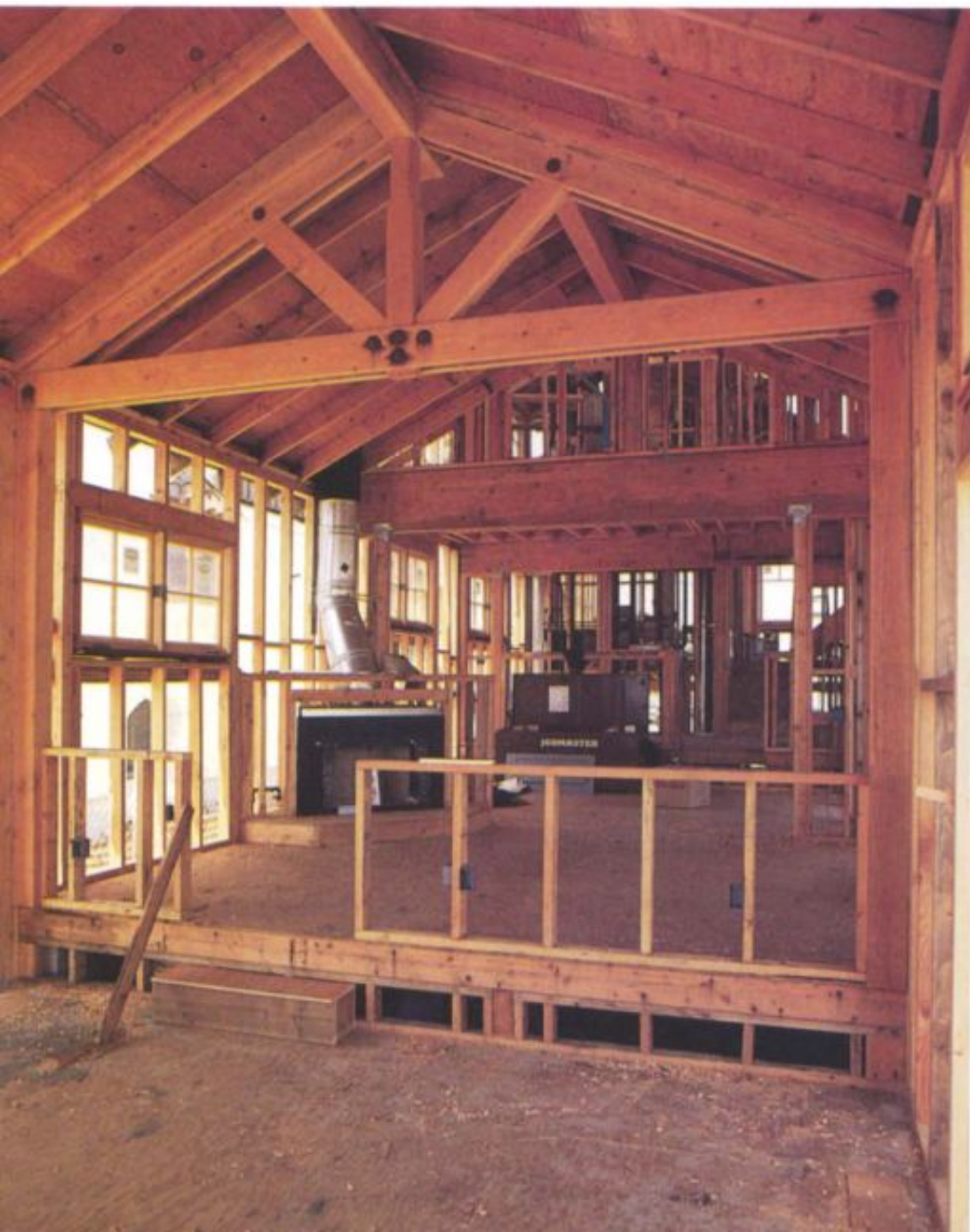
Framing, plain and fancy. The floors and walls for this California beach house are conventional 2x framing (above), except for purlins that extend the top plates of the long exterior walls. These 6x6s are supported with Craftsman-style knee braces. The concrete-block foundation walls were laid up flush with the wood framing and later plastered as a continuous surface. The king-post truss that separates the family room from the living room (below), combines wood joinery and metal fasteners in a design that's both handcrafted and practical. The tops of the two posts are tenoned to form seats for the bottom chords, and the king post and web members are also tenoned on both ends where they are sandwiched between the double chords.
