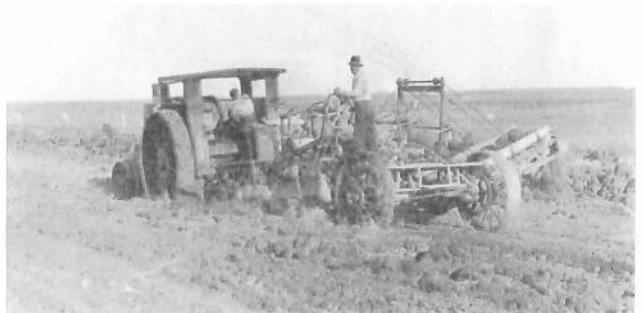
Glenn Copeland on elevating grader. Harry Copeland driving Avery 40-80, 1918 or 1919.
