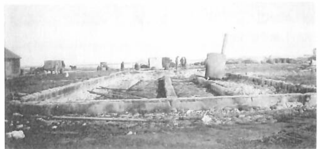
After hall burnt.
