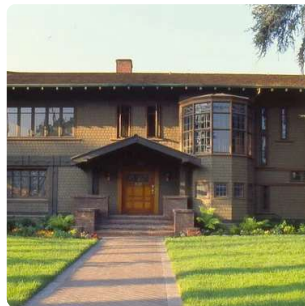
First phase restoration
