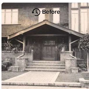
1906 entry and terrace
