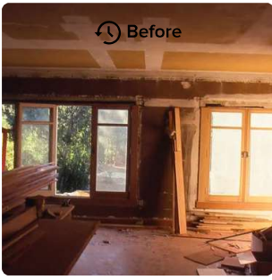
Living room during restoration
