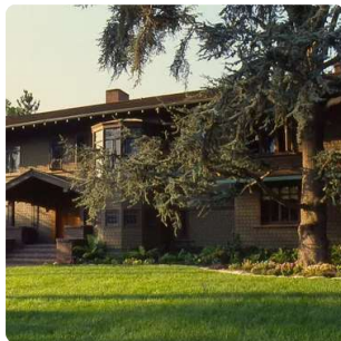
First phase restoration
