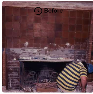
Original fireplace uncovered
