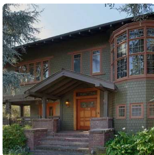
Entry and covered terrace restored
